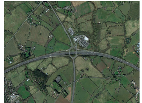
M42 Junction 2 Redditch
